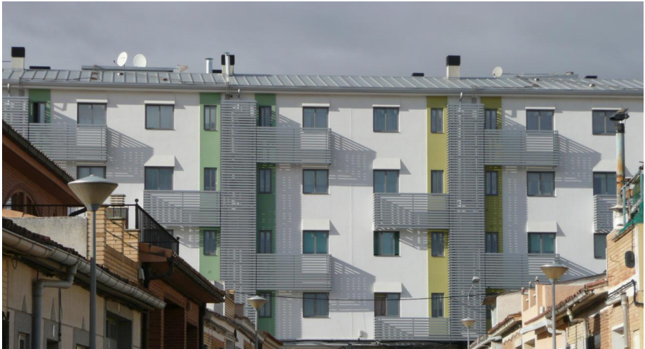
Figure 14: Some of the buildings renovated through the Lourdes Renove project.
